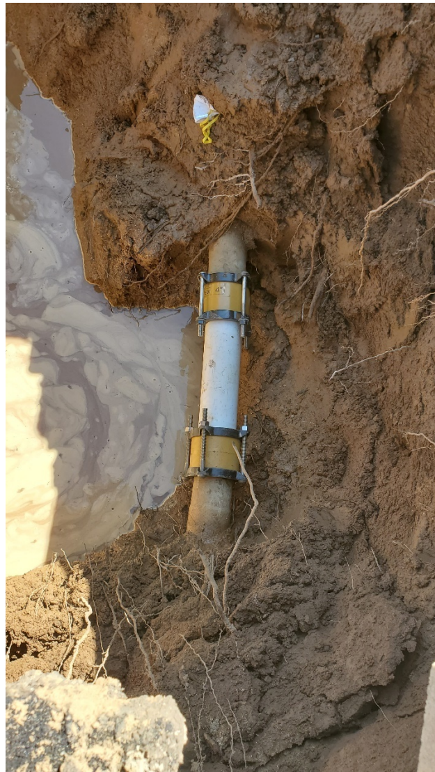
Completed repair on Mesaloo Lane water main
