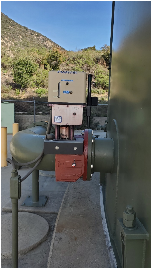
Completed replacement of butterfly valve at West Tank
