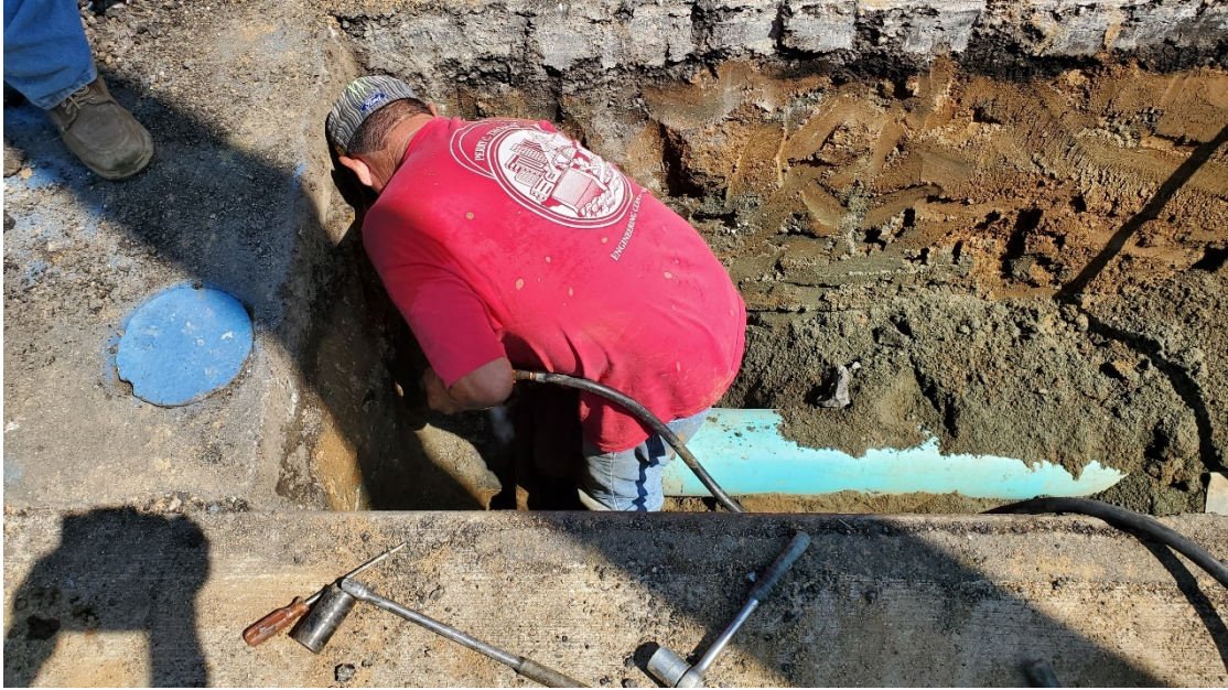
Leak repair on Villa Knolls Drive water main
