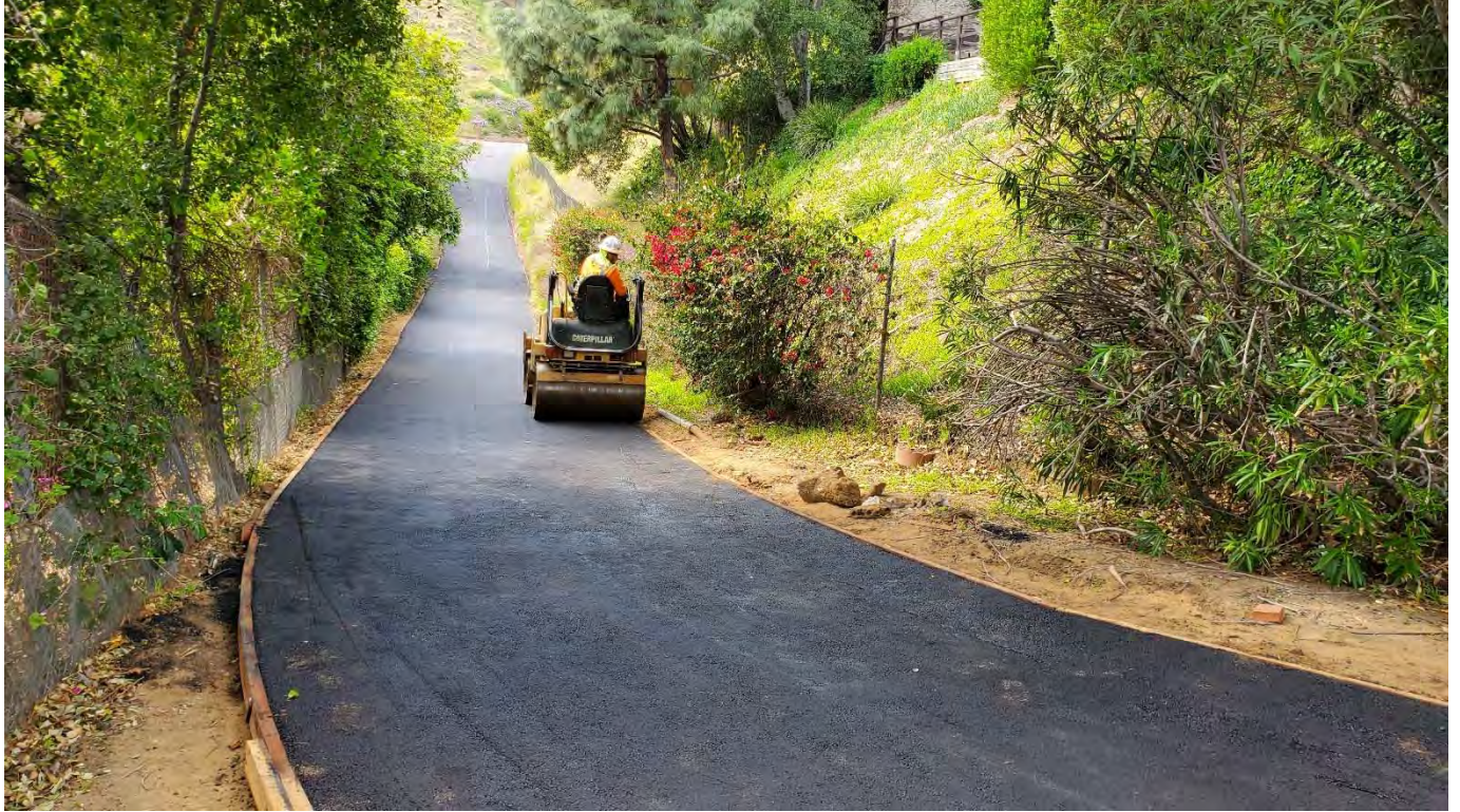
Office driveway was replaced and widened
