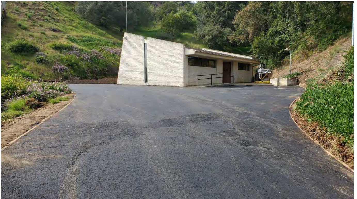
Parking area was expanded
