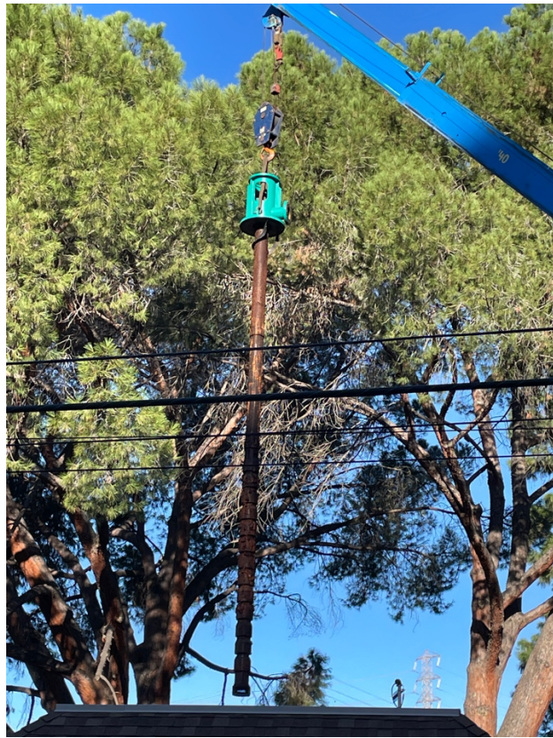
New Eucalyptus Booster #3 Pump and Motor Installed on 11/29/23
