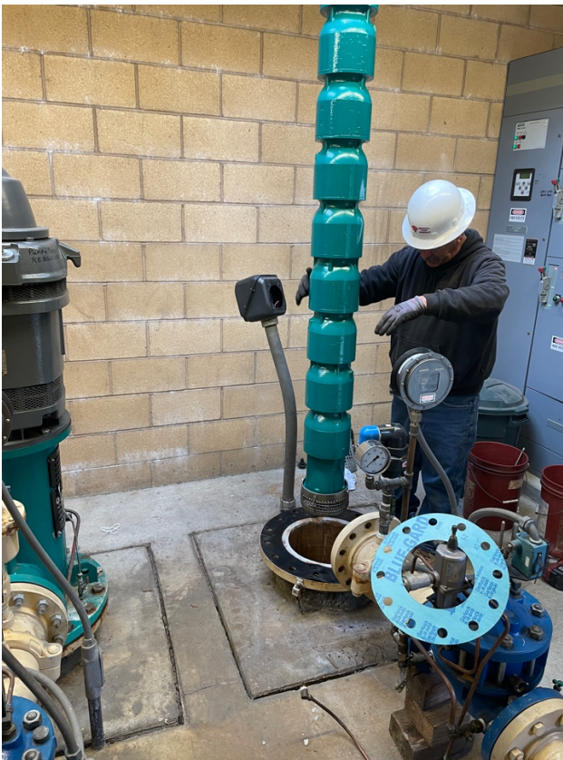
New Eucalyptus Booster #3 Pump and Motor Installed on 11/29/23
