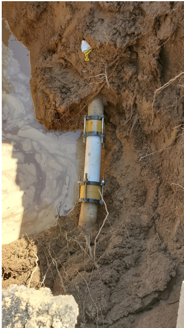
Completed repair on Mesaloe Lane water main
