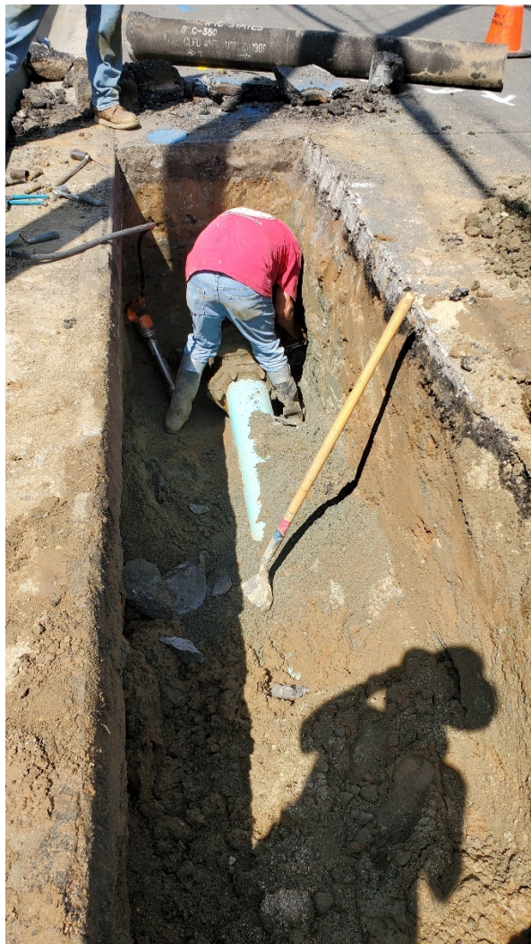
Leak repair on Villa Knolls Drive water main
