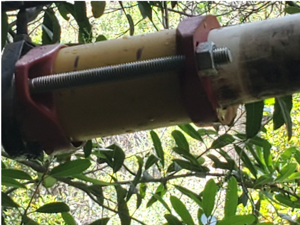
Completed repair of the House Tunnel supply line
