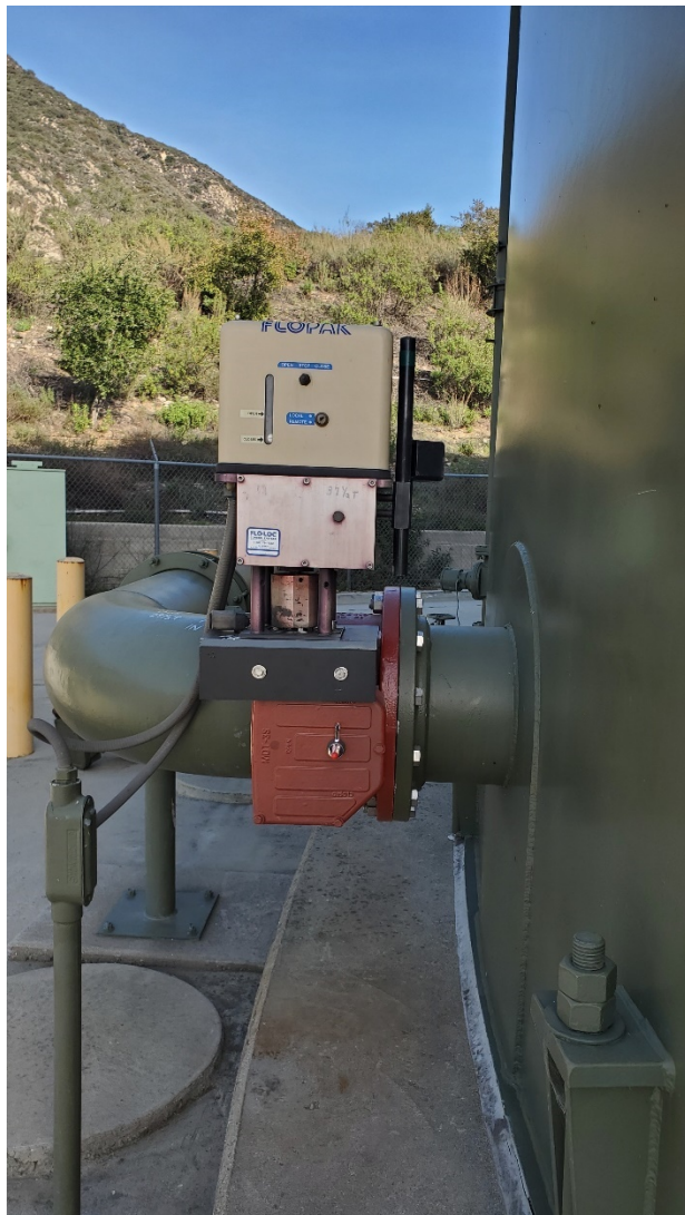
Completed replacement of butterfly valve at West Tank
