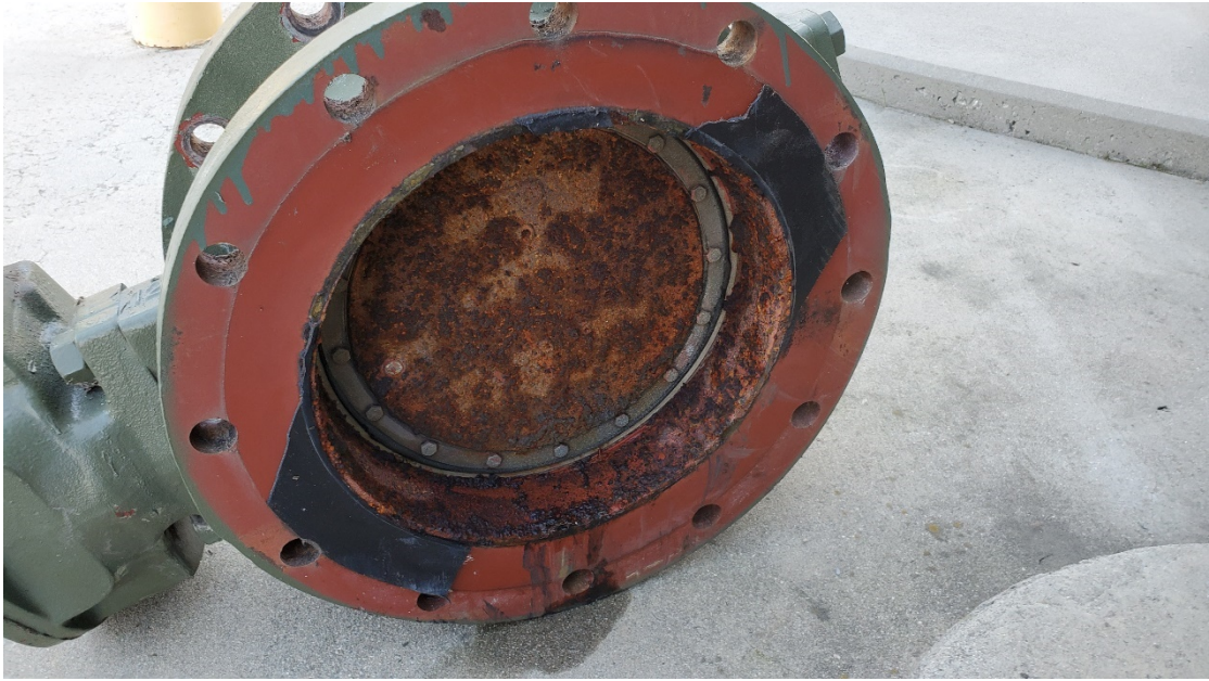
Replacement of leaking butterfly valve at West Tank
