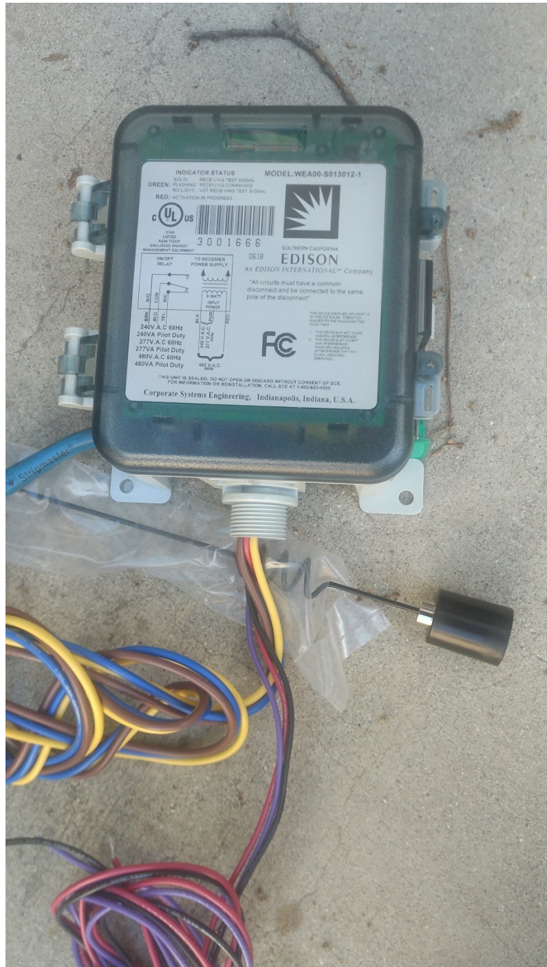
Installation of new radios at three sites for the agriculture and pumping interruption (API) rate reduction program
