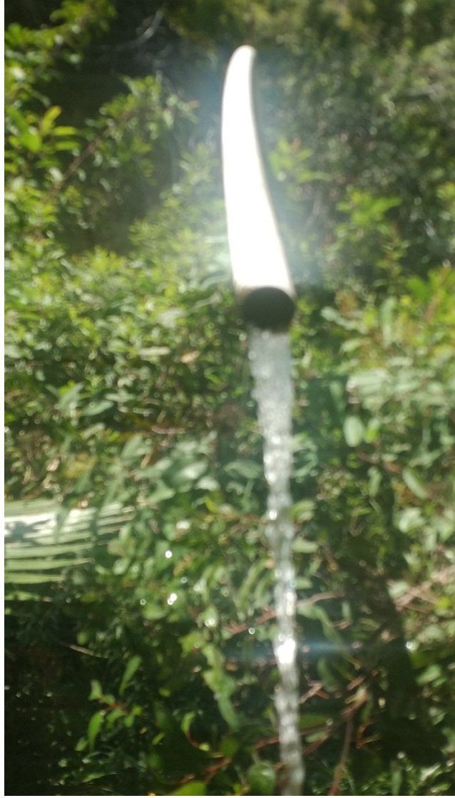
Broken House Tunnel supply line discharging water into the canyon
