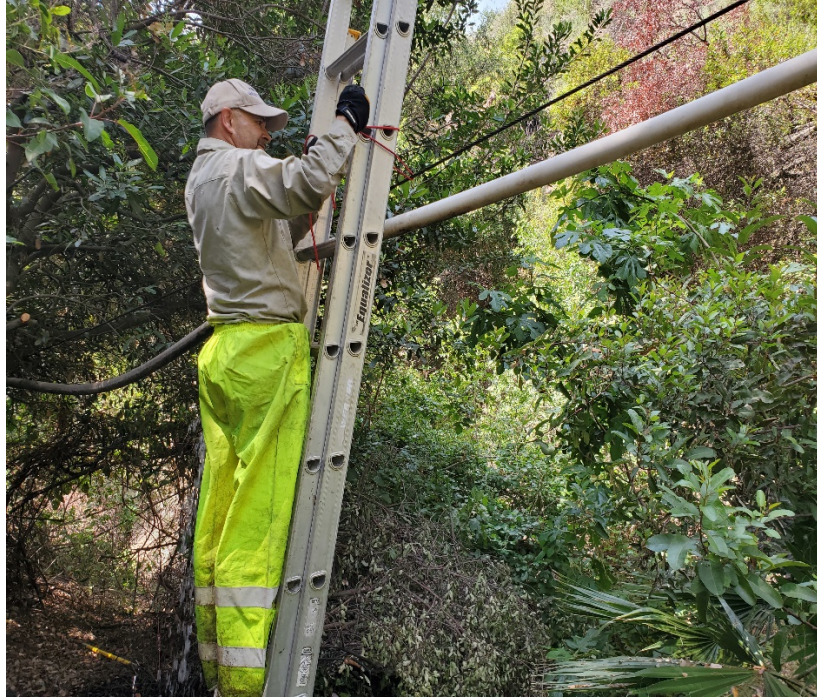
Preparation for the repair of the House Tunnel supply line
