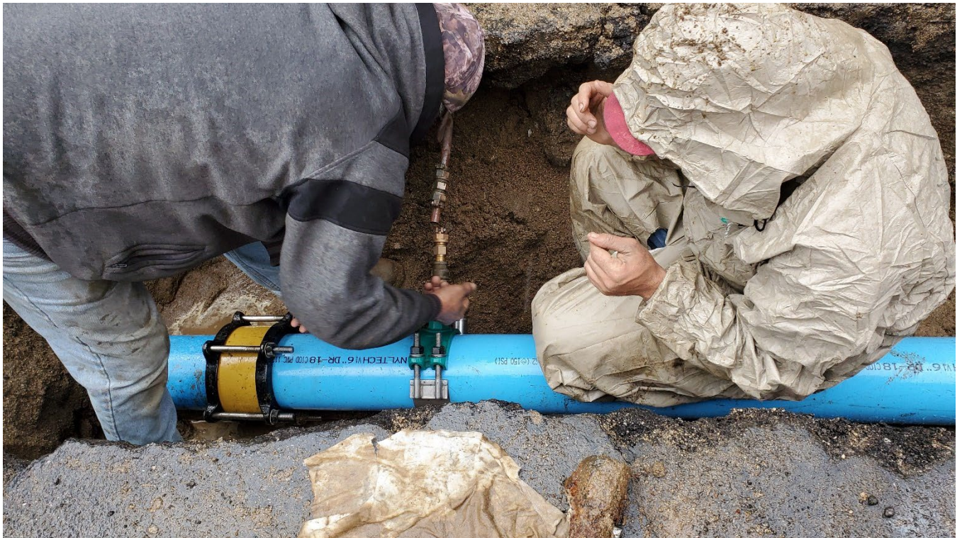
Water main repair in Pasadena Glen.
