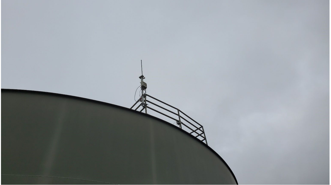
Communications equipment was installed at three District Locations.
