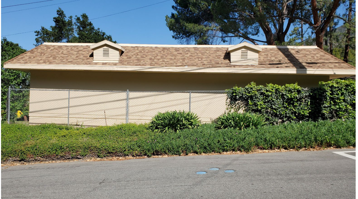
Eucalyptus Reservoir and Pump House were repainted.
