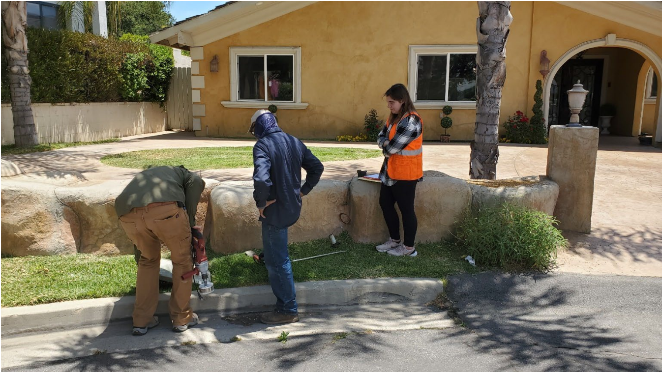
Contractor and District crew install advance metering equipment. Item 6b - Page 9
